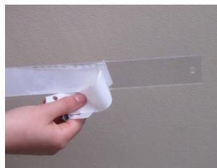
2. Remove membrane partially on both sides of the strip.
