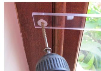
3. Install the second screw at a slight angle away from the middle of the window.
